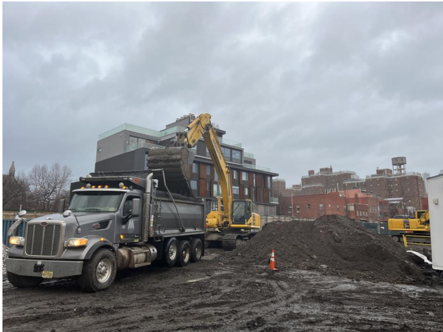
Photo 2: Kingdom exporting non-hazardous soil in a permitted tri-axle truck for off-site disposal from Society Brooklyn (facing north)
