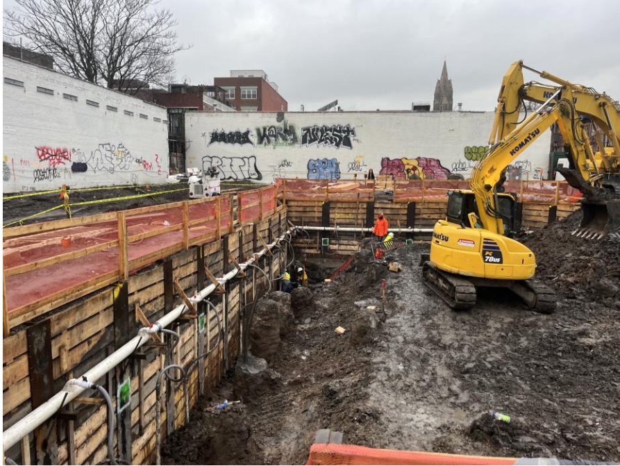
Photo 1: Kingdom excavating for the future cellar in the northern part of Sackett Place (facing southwest)
