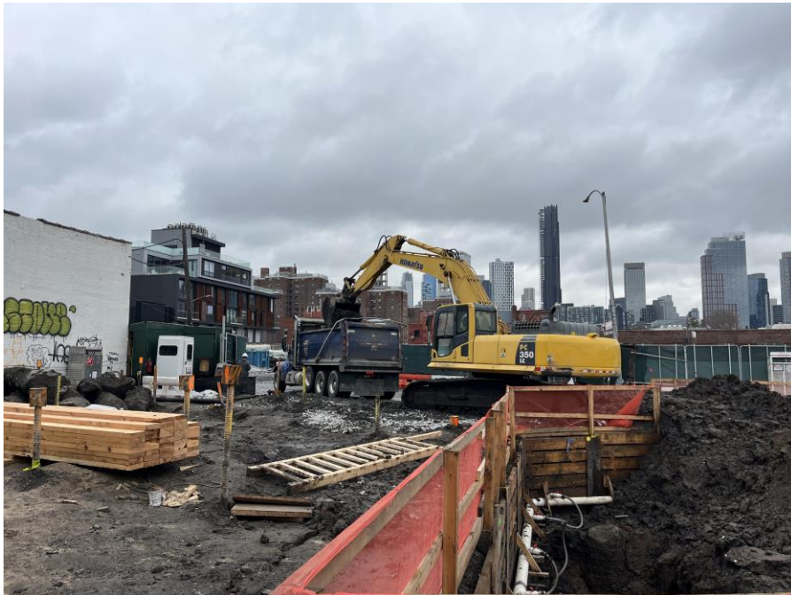
Photo 2: Kingdom exporting non-hazardous soil in a permitted tri-axle truck for off-site disposal from Sackett Place (facing north)
