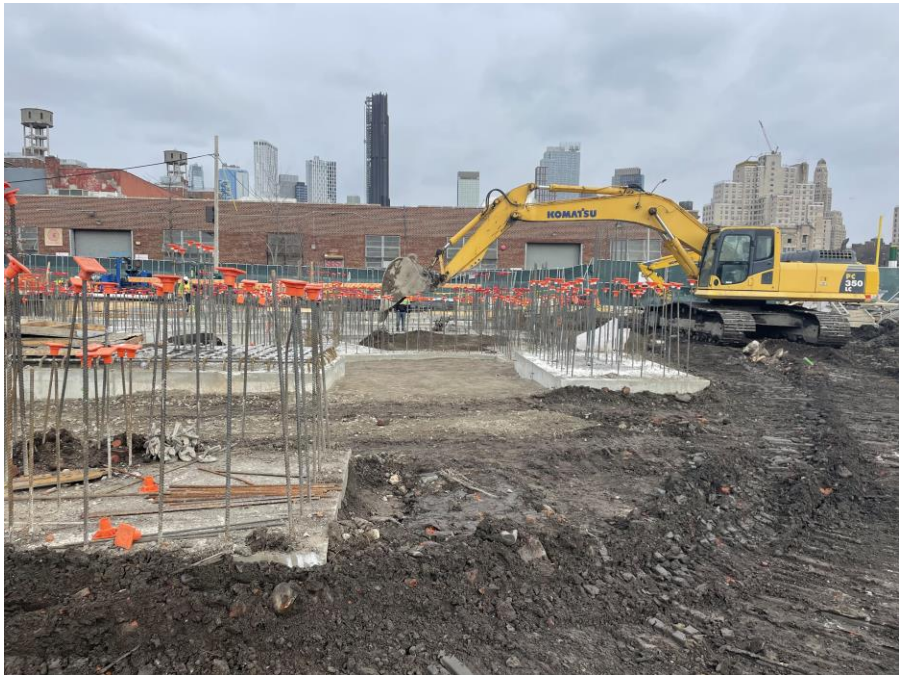
Photo 1: Kingdom backfilling around structural pile caps in the northeastern part of Society Brooklyn. (facing northwest)
