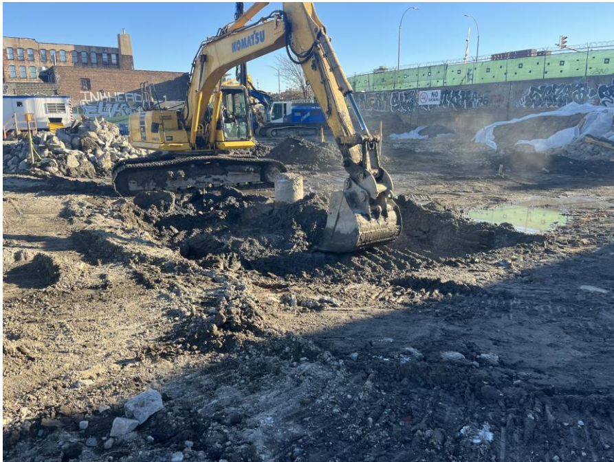
Photo 2: Kingdom excavating within Remedial Excavation Area No. 4 in the southern part of Sackett Place (facing southeast).
