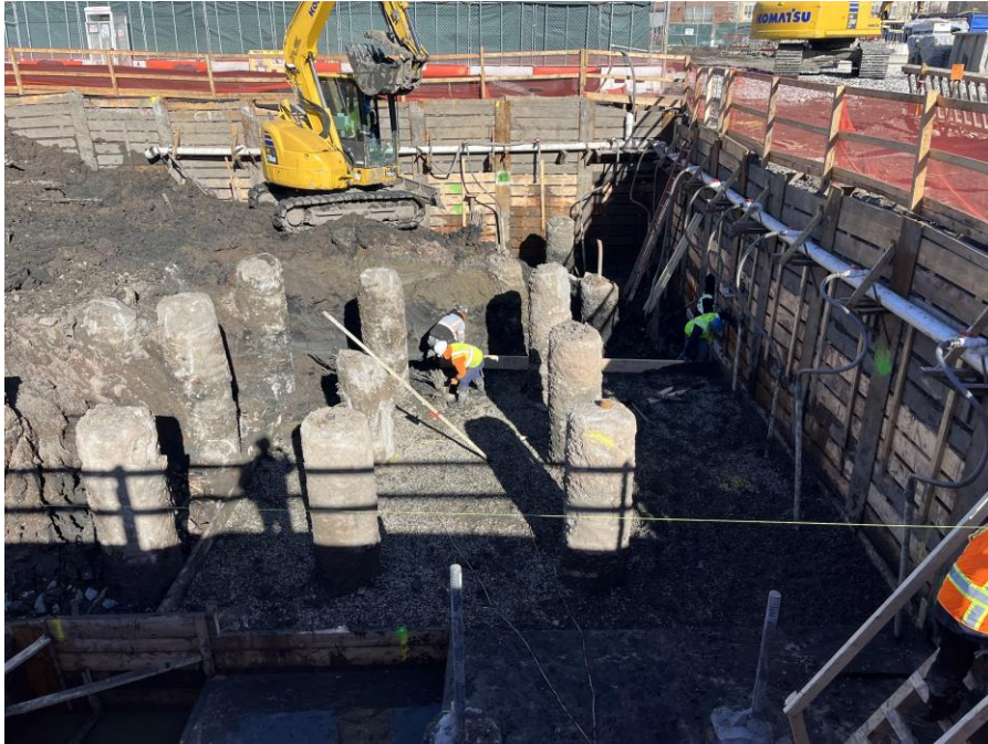
Photo 1: Kingdom installing formwork for structural pile caps and a cellar-level mud slab in the northern part of Sackett Place (facing north)
