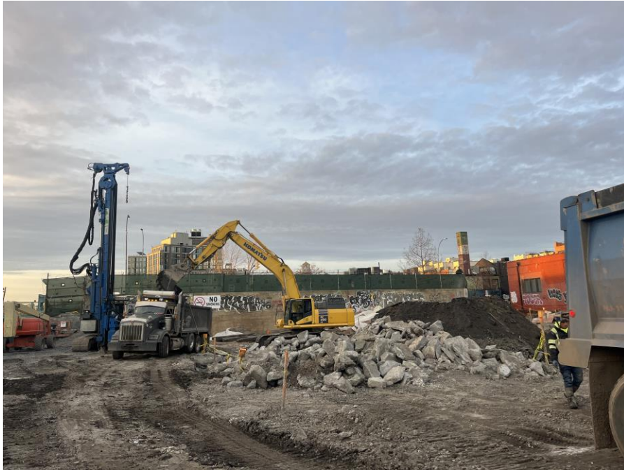
Photo 1: Kingdom exporting non-hazardous soil in a permitted tri-axle truck for off-site disposal from Remedial Excavation No. 4 in the southern part of Sackett Place (facing south)
