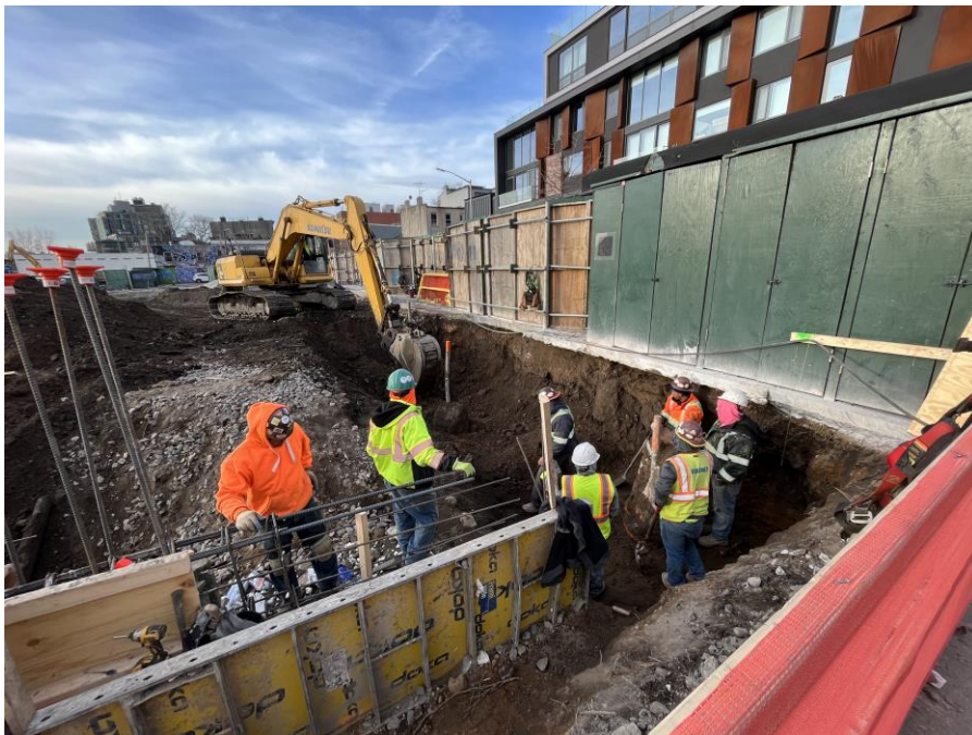
Photo 2: Kingdom excavating to install formwork in the northwestern part of Society Brooklyn (facing southwest)
