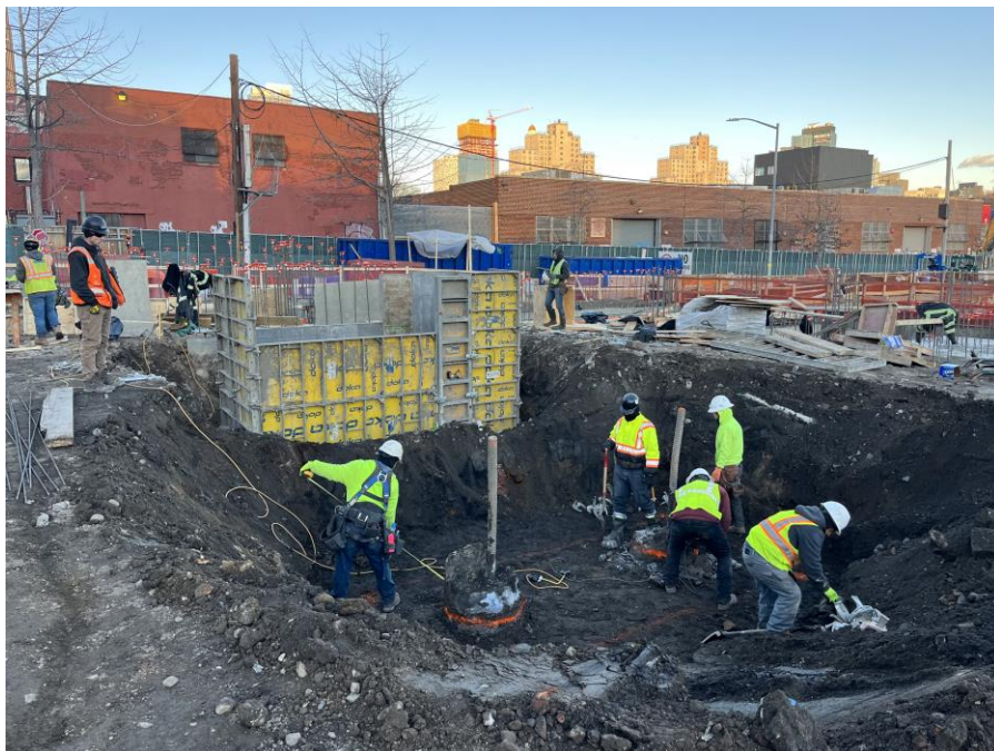
Photo 2: Kingdom excavating to install structural pile cap formwork in the northwestern part of Society Brooklyn (facing northeast)
