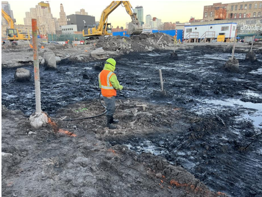
Photo 1: Kingdom applying Petrofix reagent to the base and sidewalls of Remedial Excavation Area No. 4 in the southern part of Sackett Place (facing northeast)
