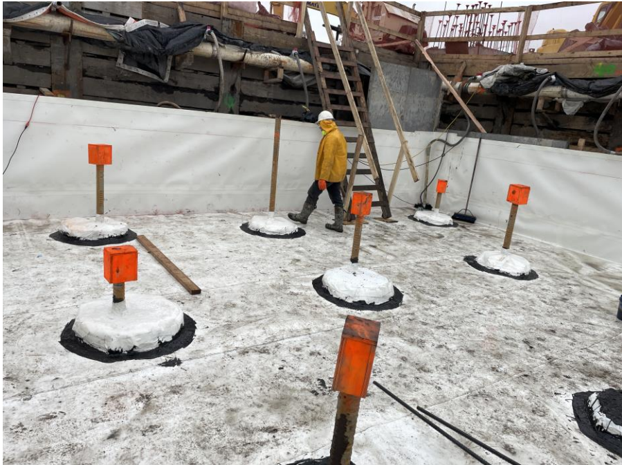
Photo 2: Kingdom installing a waterproofing/vapor barrier membrane in the southern part of Society Brooklyn (facing northeast)
