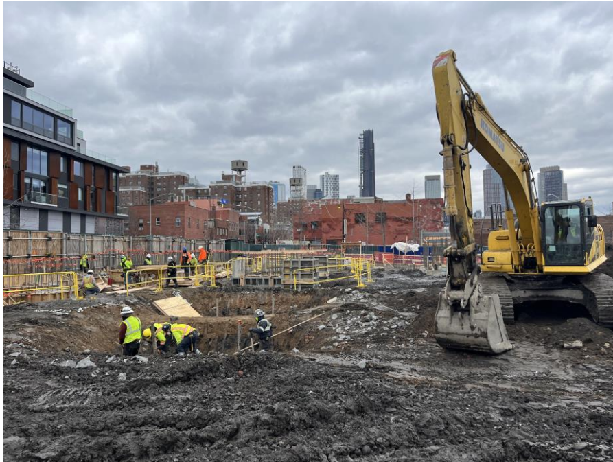
Photo 1: Kingdom excavating to install structural pile cap formwork in the western part of Society Brooklyn (facing north)
