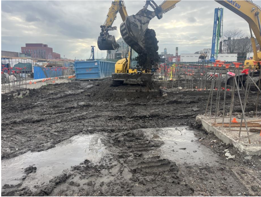
Photo 1: Kingdom backfilling to create a level working surface in the eastern part of Society Brooklyn (facing south)
