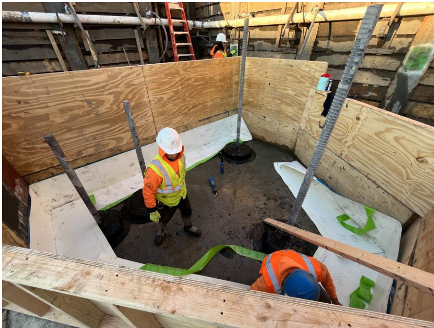
Photo 2: Kingdom installing a waterproofing/vapor barrier membrane in the northern part of Sackett Place (facing northwest)
