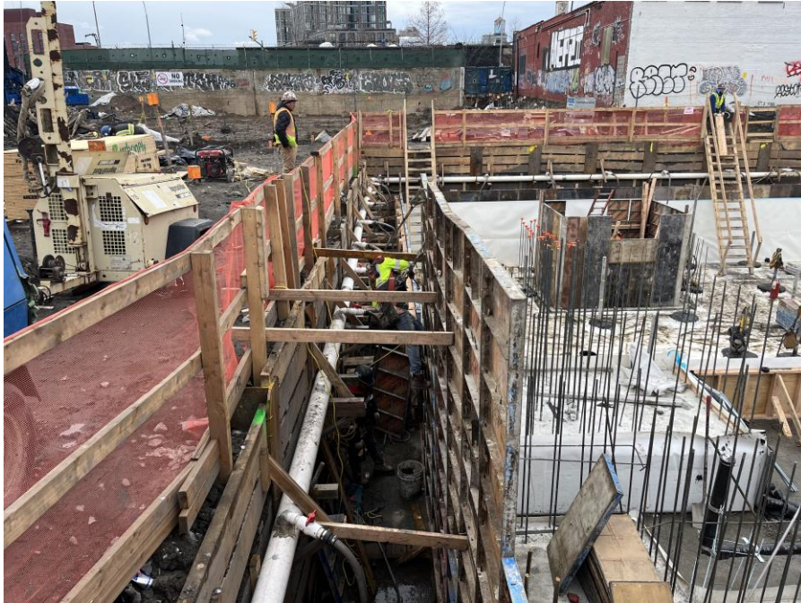
Photo 1: Kingdom installing foundation wall formwork in the northern part of Sackett Place (facing south)
