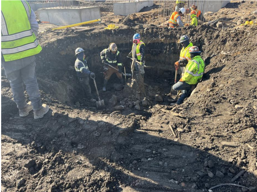
Photo 1: Kingdom excavating to install foundation pile formwork in the southwestern part of Society Brooklyn (facing southwest)
