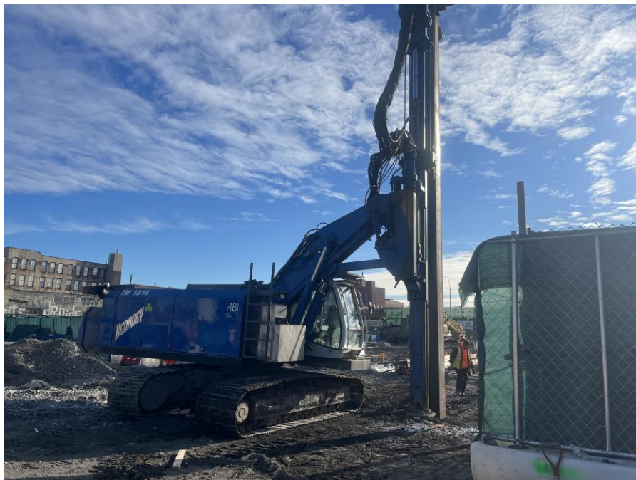
Photo 2: Kingdom installing soldier piles for the SOE in the northeastern part of Sackett Place (facing southeast)
