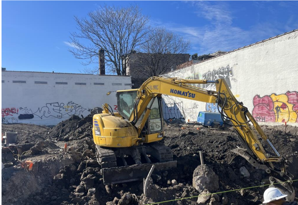
Photo 1: Kingdom excavating to install formwork in the northwestern part of Sackett Place (facing south)
