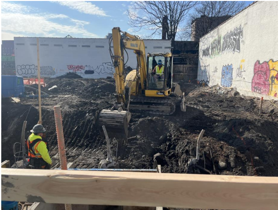
Photo 1: Kingdom excavating to install formwork in the northwestern part of Sackett Place (facing south)
