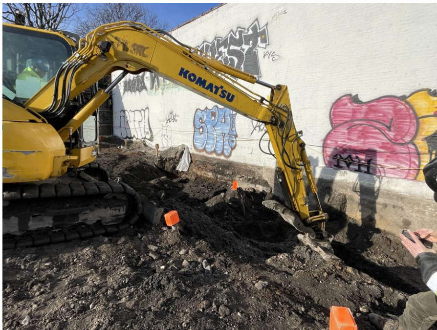
Photo 1: Kingdom excavating to remove petroleum-impacted soil/fill from beneath the former UST in the northwestern part of Sackett Place (facing southwest)
