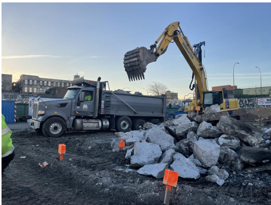
Photo 2: Kingdom loading a permitted tri-axle truck with C&D debris for off-site disposal from Sackett Place (facing southeast)
