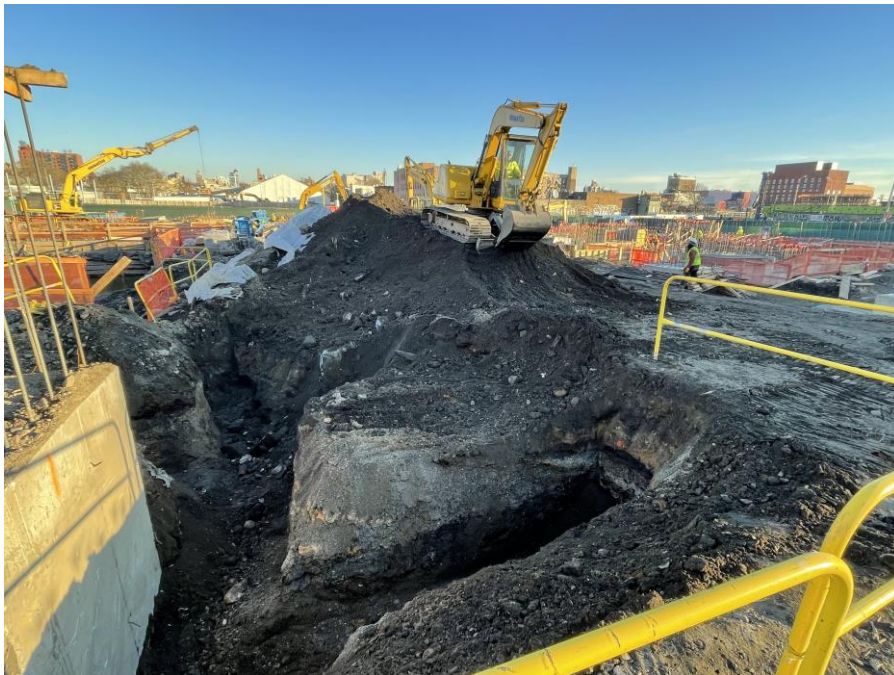
Photo 2: Kingdom excavating to install formwork in the northwestern part of Society Brooklyn (facing southeast)
