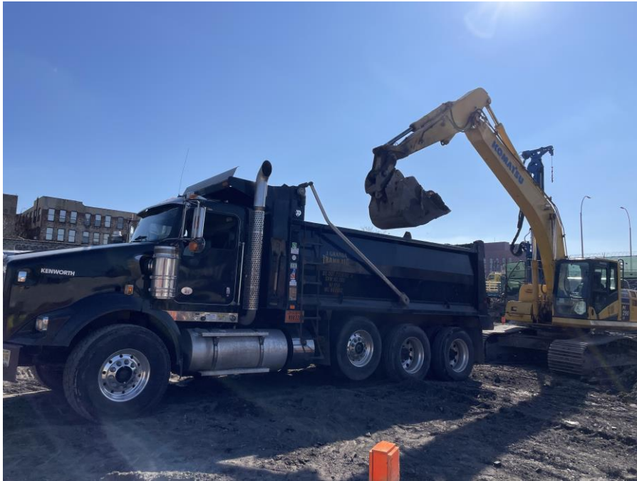
Photo 1: Kingdom exporting non-hazardous soil into a permitted tri-axle truck for off-site disposal from Sackett Place (facing southeast)
