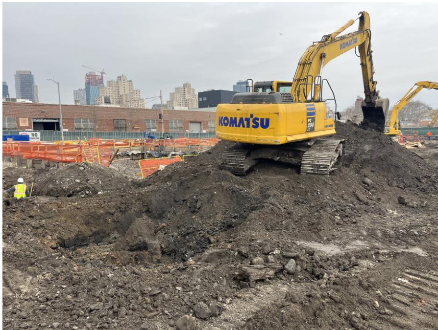
Photo 2: Kingdom excavating to install formwork in the central part of Society Brooklyn (facing northeast)
