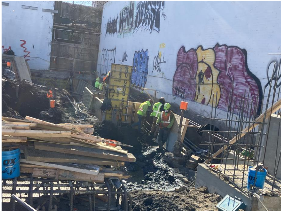
Photo 1: Kingdom applying Petrofix reagent to the base and sidewalls of the form UST excavation in the northwestern part of Sackett Place (facing southwest)
