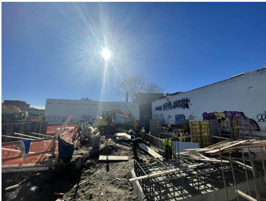
Photo 2: Kingdom excavating to install pile cap formwork in the western part of Sackett Place (facing southwest)
