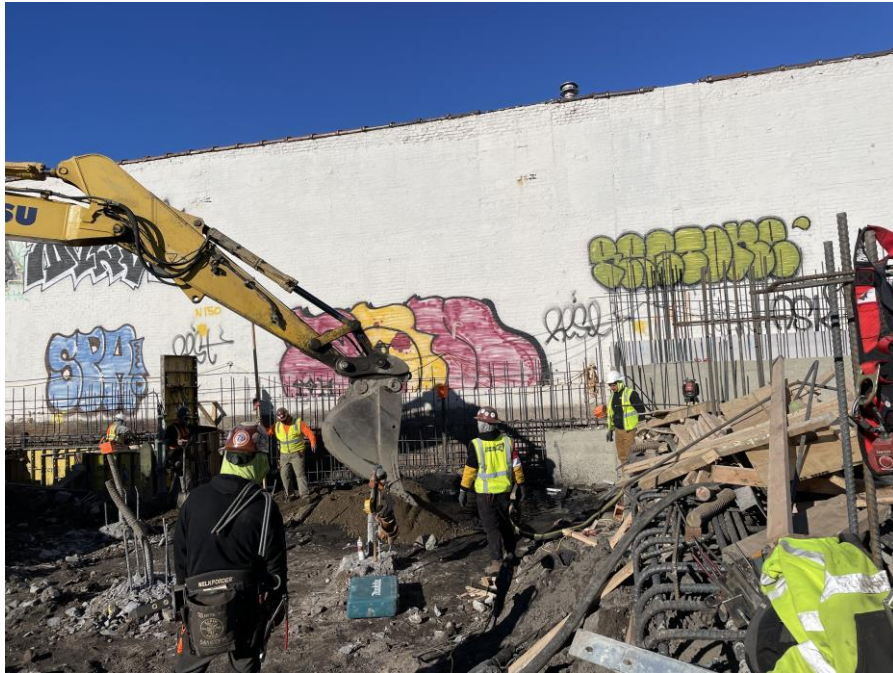
Photo 1: Kingdom backfilling a former UST excavation following treatment with Petrofix on 2/10 in the northwestern part of Sackett Place (facing west)
