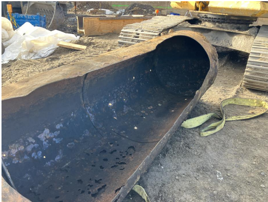
Photo 2: View of cleaned UST prior to off-site disposal (facing south)
