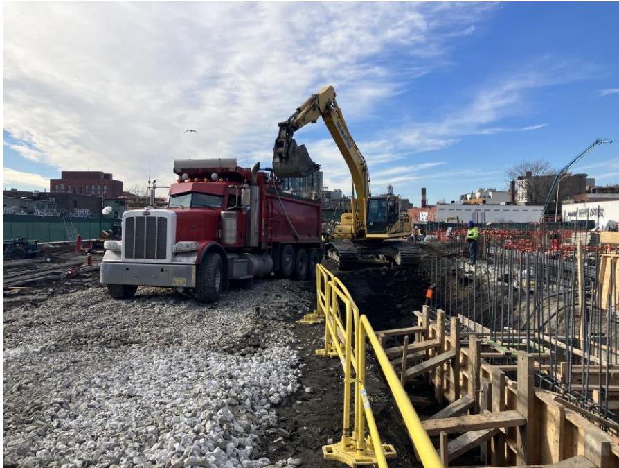
Photo 1: Kingdom exporting non-hazardous soil in a permitted tri-axle truck for off-site disposal from Society Brooklyn (facing southwest)
