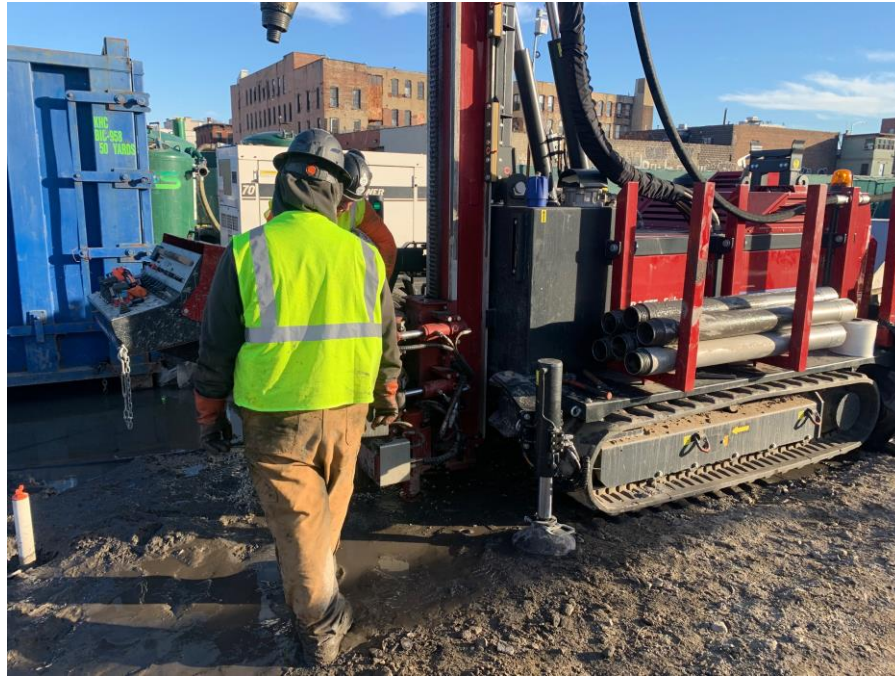
Photo 3: Costal advancing soil boring SB39 in the southeastern part of Society Brooklyn (facing southeast)
