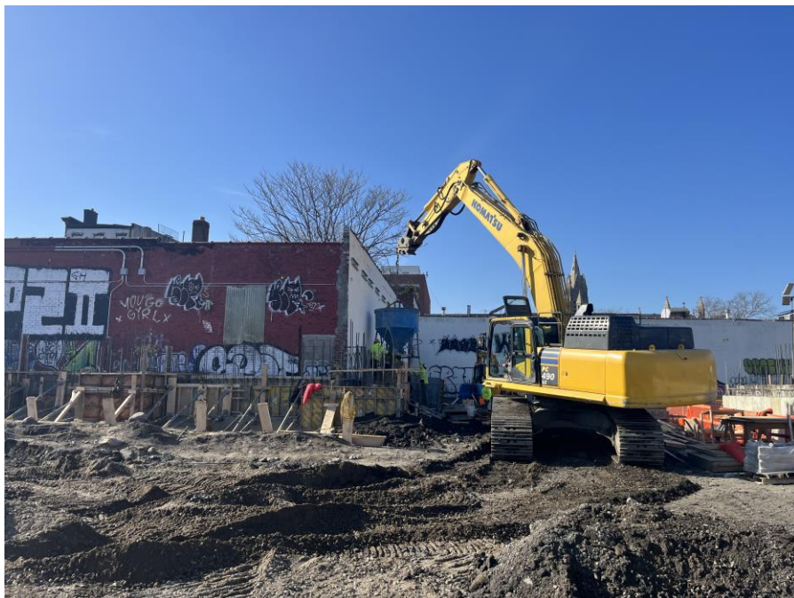
Photo 2: Kingdom placing concrete for structural pile caps in the western part of Sackett Place (facing west)
