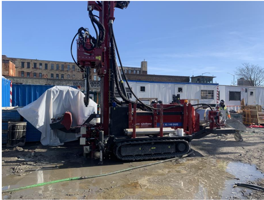
Photo 3: Coastal preparing to advance soil boring SB40A in the northeastern part of Sackett Place (facing southeast)
