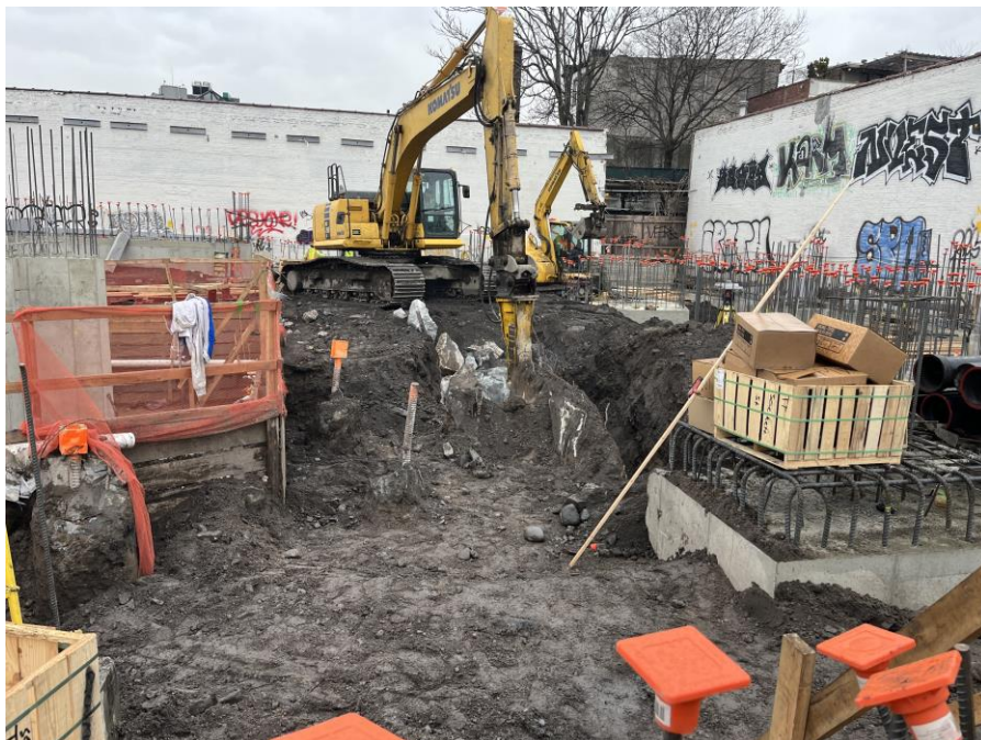
Photo 2: Kingdom demolishing historical concrete foundation elements to install structural pile caps in the northwestern part of Sackett Place (facing south)
