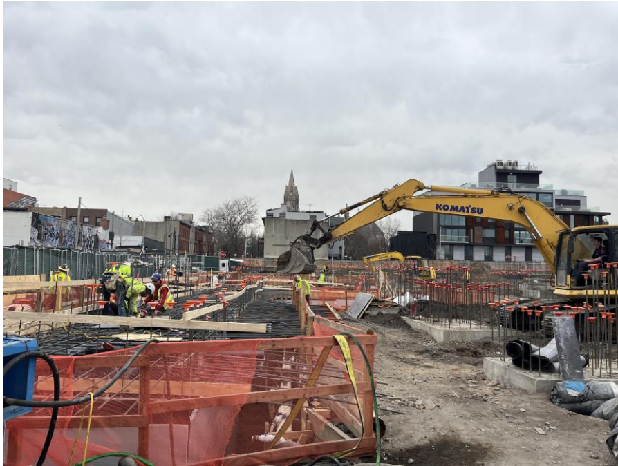
Photo 1: Kingdom backfilling around cellular formwork in the southern part of Society Brooklyn (facing west)
