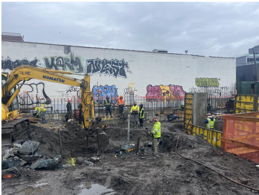
Photo 2: Kingdom excavating to install formwork in the northwestern part of Sackett Place (facing west)
