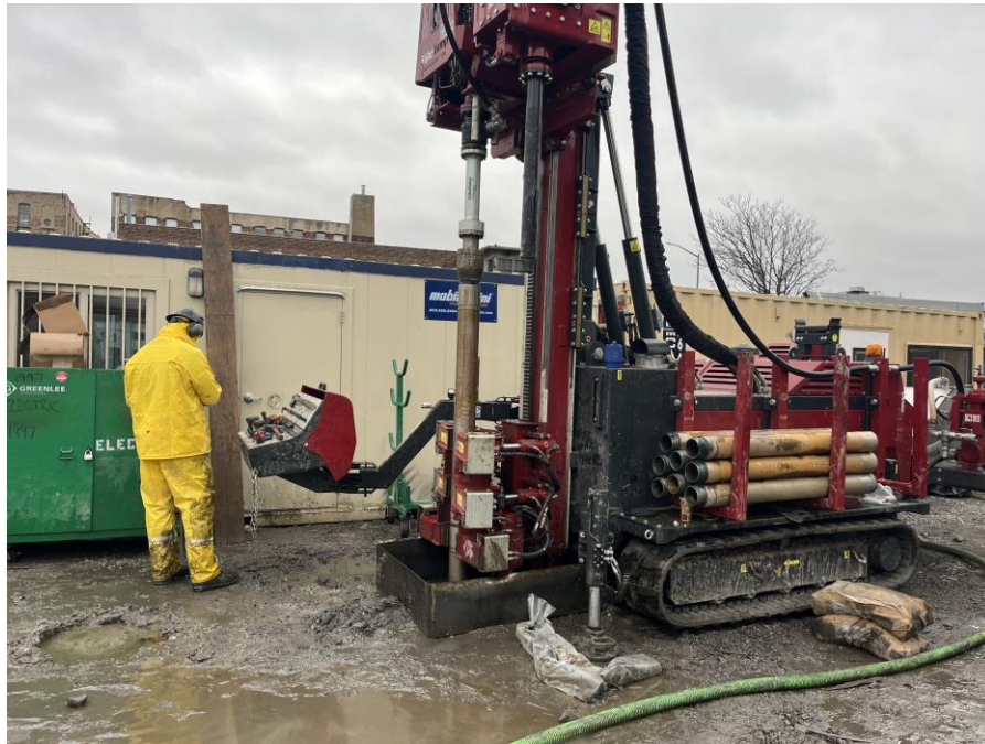
Photo 3: Coastal advancing soil boring SB41 in the southeastern part of Sackett Place (facing east)
