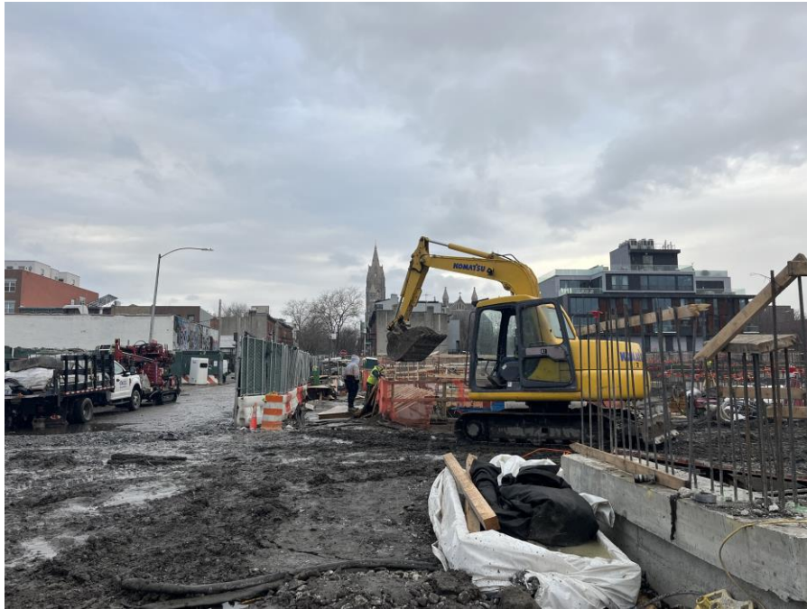
Photo 1: Kingdom backfilling around cellar wall formwork in the southern part of Society Brooklyn (facing west)
