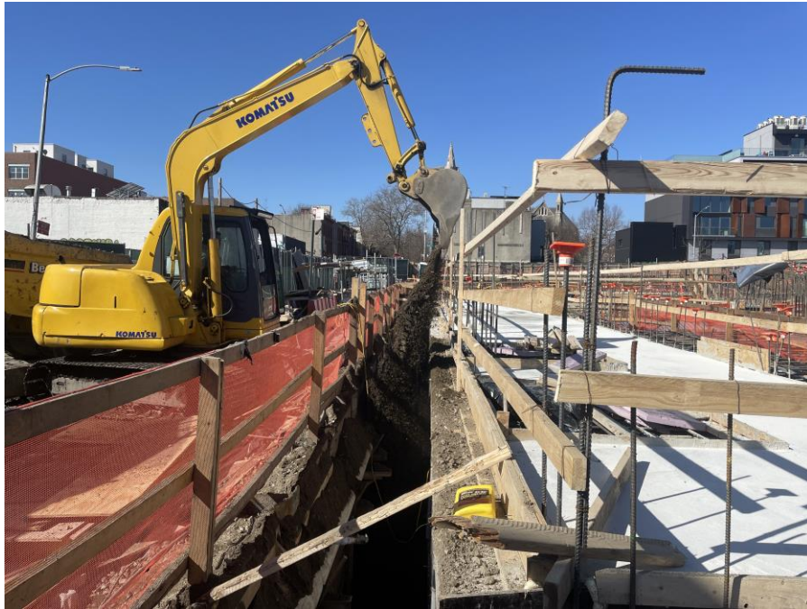
Photo 1: Kingdom backfilling around the cellar wall in the southern part of Society Brooklyn (facing west)
