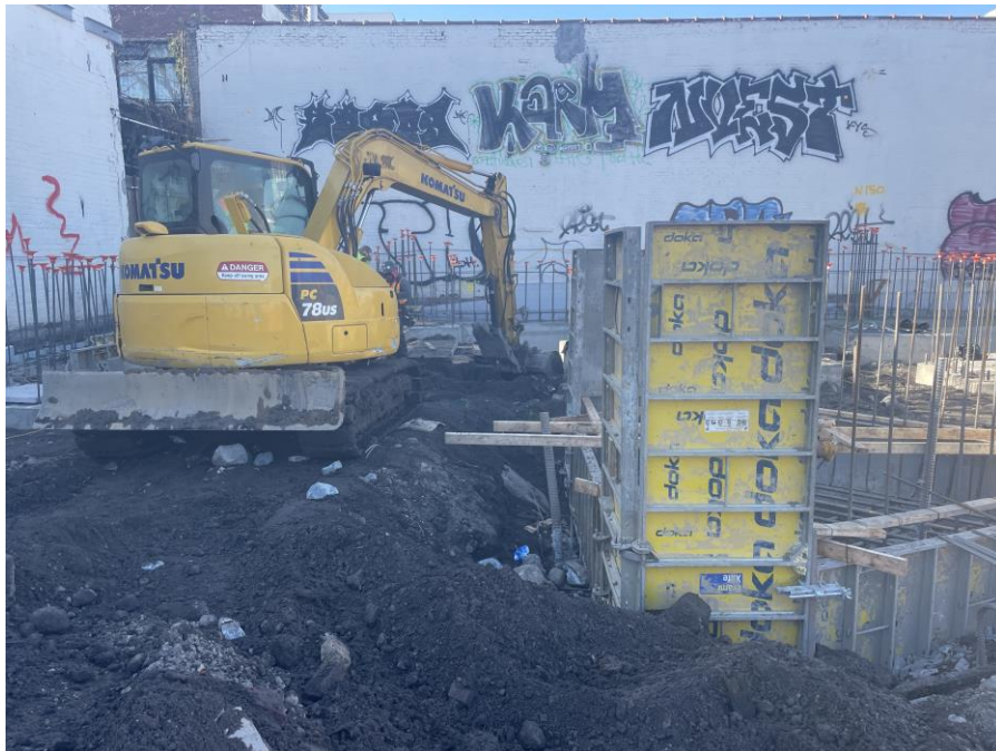
Photo 2: Kingdom excavating to install structural pile caps in the northwestern part of Sackett Place (facing west)
