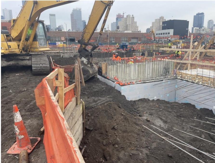
Photo 1: Kingdom backfilling around the cellar wall in the southern part of Society Brooklyn (facing northeast)
