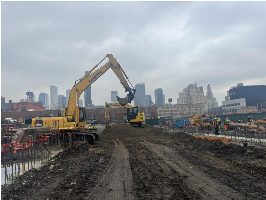
Photo 2: Kingdom excavating in the northern part of Society Brooklyn for off-site disposal (facing southeast)
