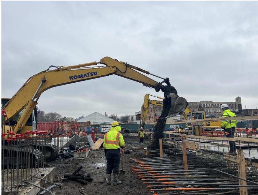
Photo 1: Kingdom backfilling around the cellar wall in the southern part of Society Brooklyn (facing south)
