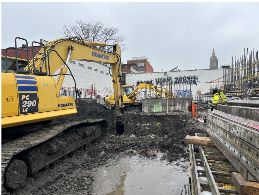
Photo 2: Kingdom excavating to install structural pile caps in the western part of Sackett Place (facing west)
