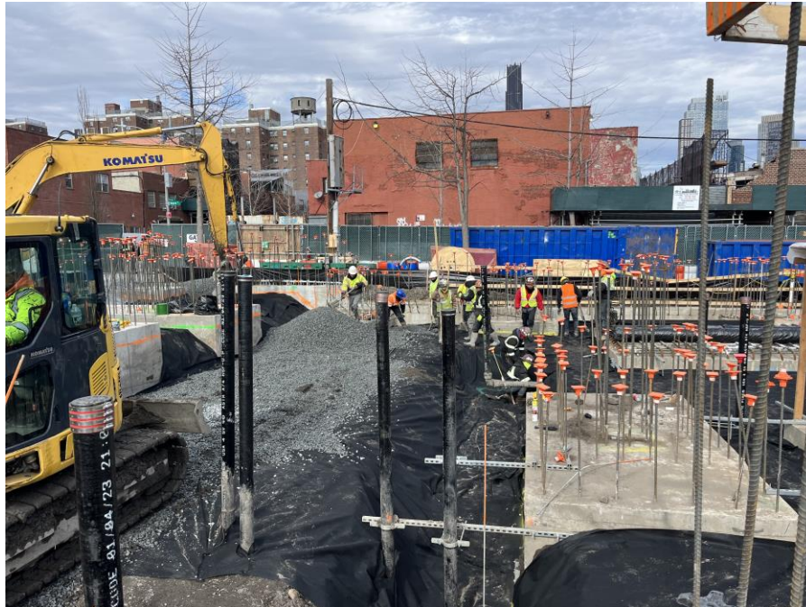
Photo 1: Kingdom backfilling with ASTM#5 stone as part of the SMD system in the northern part of Society Brooklyn (facing north)
