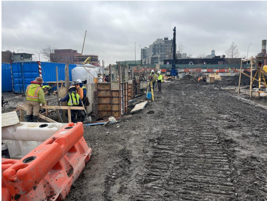
Photo 1: Kingdom installing formwork in the northeastern part of Sackett Place (facing northeast)
