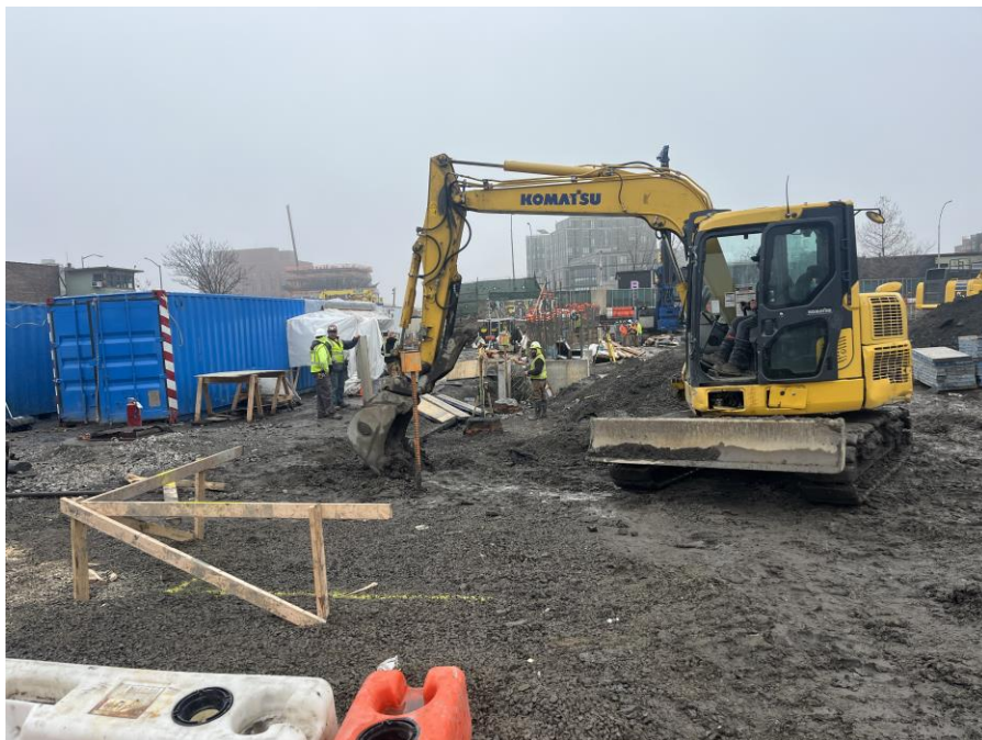
Photo 2: Kingdom excavating to install formwork in the northeastern part of Sackett Place (facing south)
