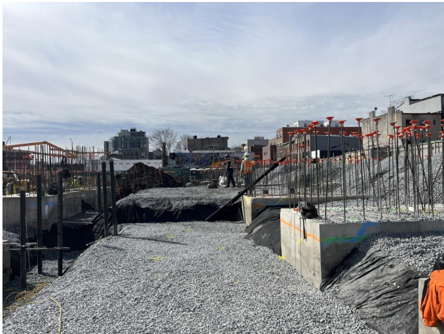
Photo 2: Kingdom placing ASTM#5 stone as a part of SMD system installation in the northern part of Society Brooklyn (facing south)
