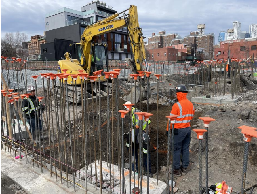
Photo 1: Kingdom excavating to install utilities in the western part of Society Brooklyn (facing northwest)
