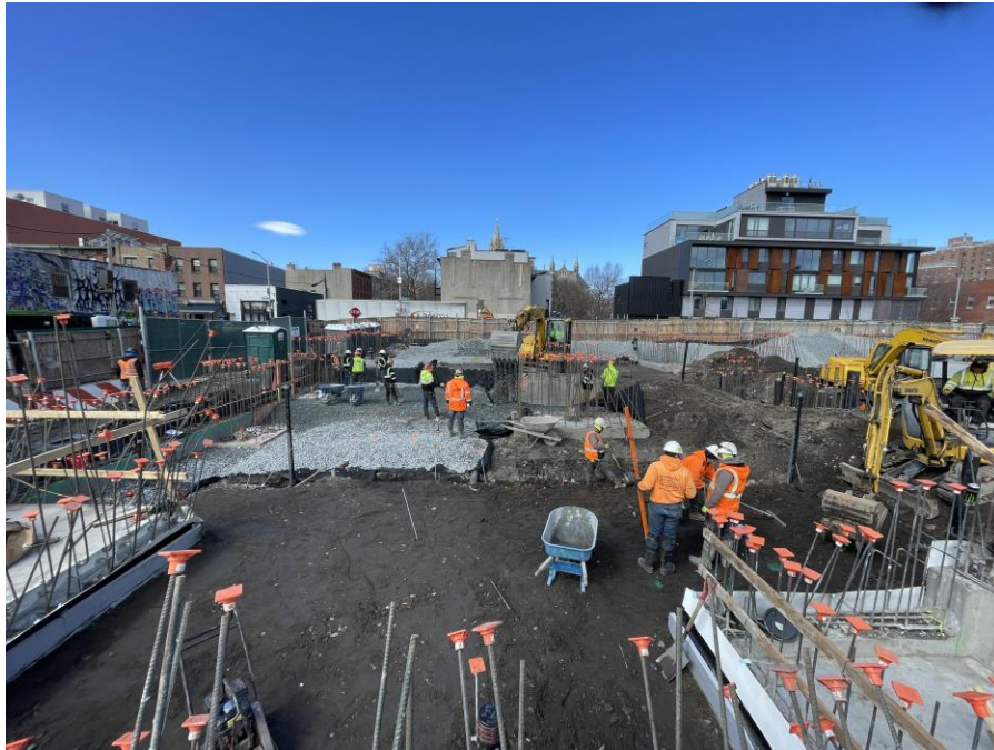
Photo 1: Kingdom grading in the southwestern part of Society Brooklyn to install SMD system components (facing west)
