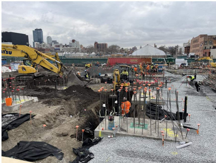
Photo 2: Kingdom excavating to install utilities in the western part of Society Brooklyn (facing east)
