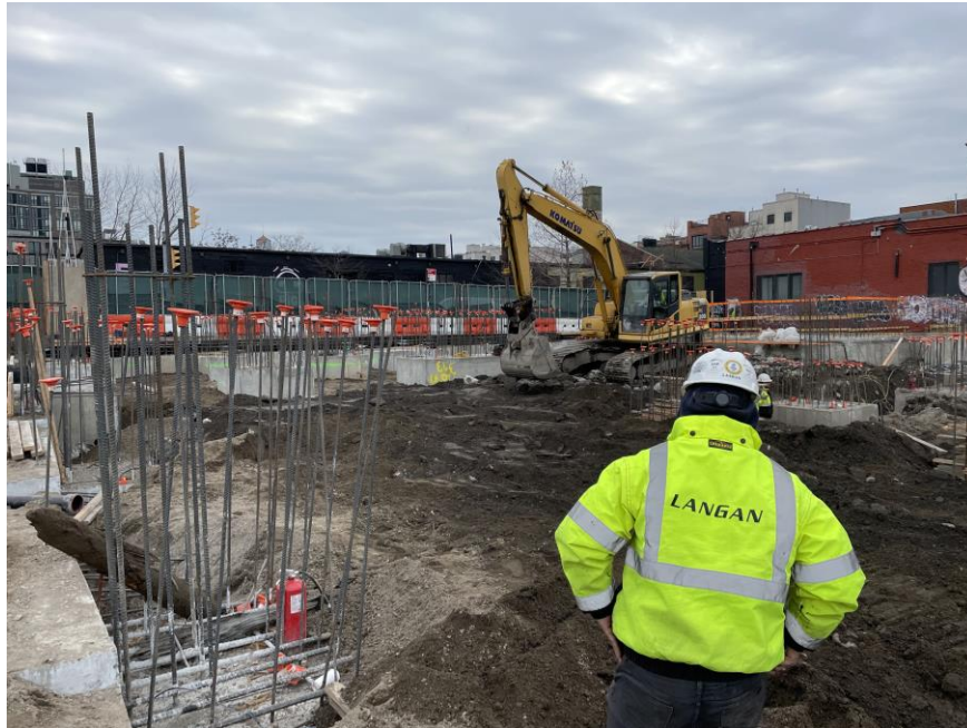
Photo 1: Kingdom backfilling around utilities in the southern part of Sackett Place (facing southwest)
