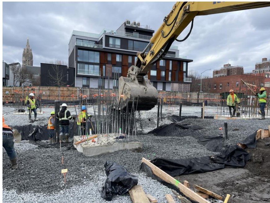
Photo 2: Kingdom installing SMD system components in the central part of Society Brooklyn (facing west)
