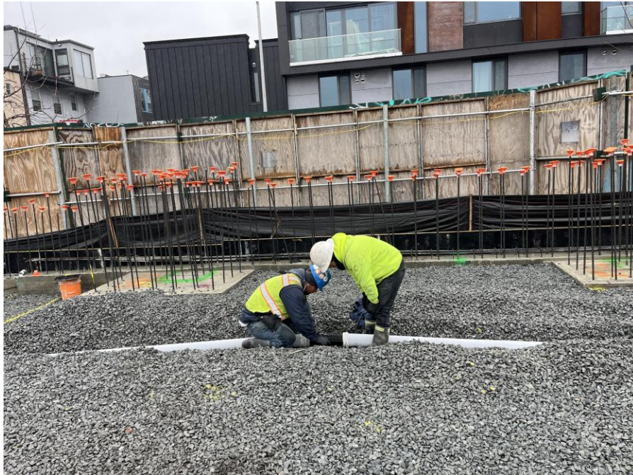
Photo 2: Kingdom using tile tape to seal the SMD system perforated piping connections in the western part of Society Building (facing west).
