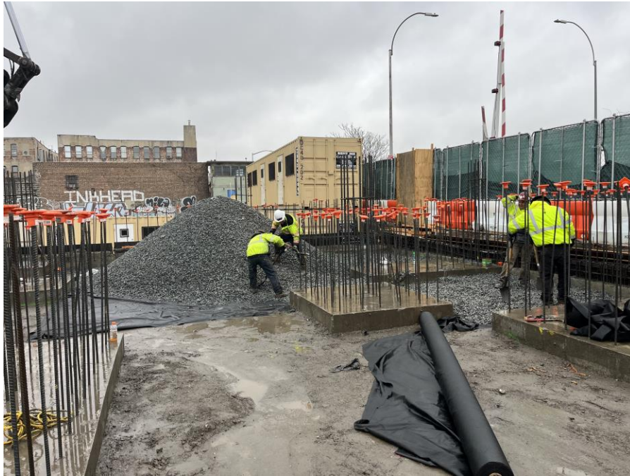
Photo 1: Kingdom installing SMD system components in the Southern part of Sackett Place (facing southeast)
