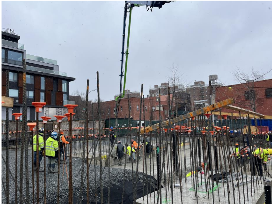
Photo 2: Kingdom placing concrete for a mud slab above the SMD system in the northwestern part of Society Brooklyn (facing north).
