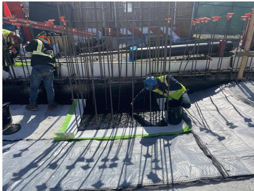
Photo 2: Kingdom installing a waterproofing/vapor barrier membrane in the western part of Society Brooklyn (southwest)
