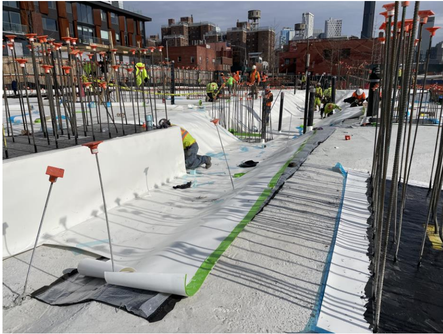
Photo 1: Kingdom installing a waterproofing/vapor barrier membrane in the western part of Society Brooklyn (facing north)
