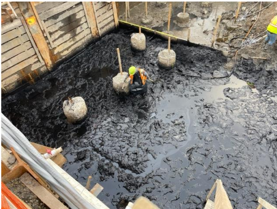
Photo 2: Kingdom applying Petrofix reagent to the base of Remedial Excavation Area No. 1 in the northern part of Society Brooklyn (facing southeast)
