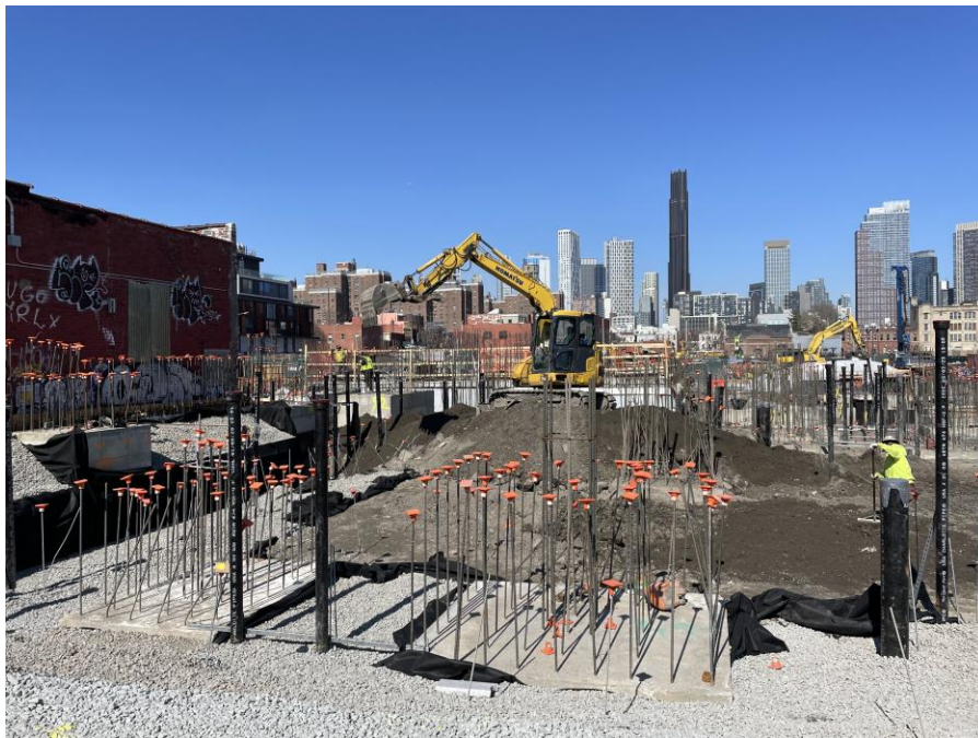
Photo 2: Kingdom grading in the southern part of Sackett Place to install components of the SMD system (facing north)
