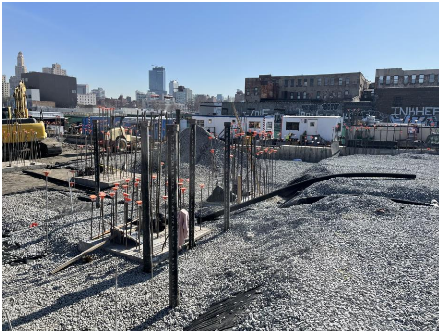
Photo 2: Kingdom backfilling with ASTM #5 stone for the SMD system in the southern part of Sackett Place (facing east)
