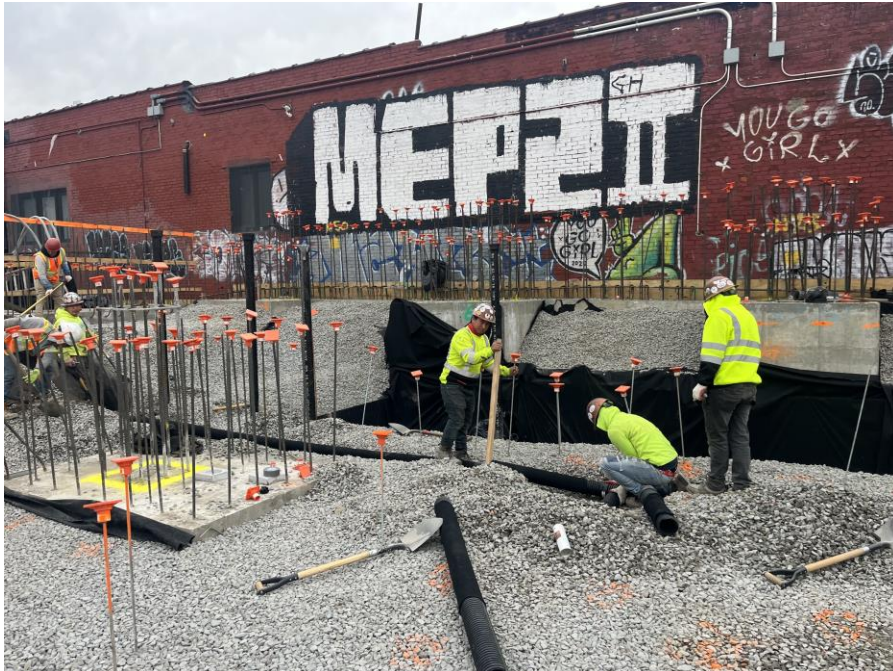
Photo 2: Kingdom installing SMD system components in the southern part of Sackett Place (facing southwest)
