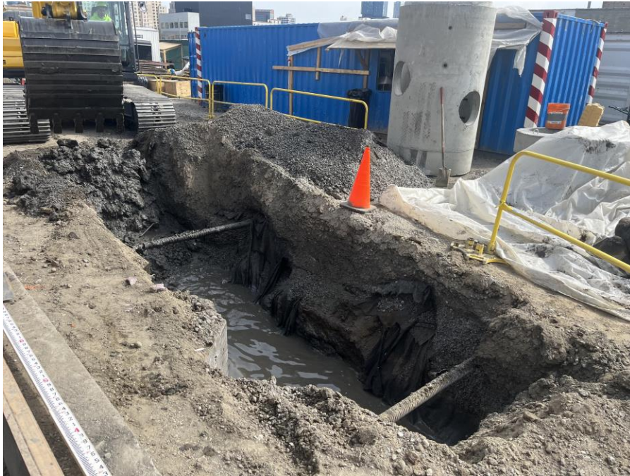
Photo 1: G&M excavating to install utilities in the eastern part of Sackett Place within the SPW (facing northeast)
