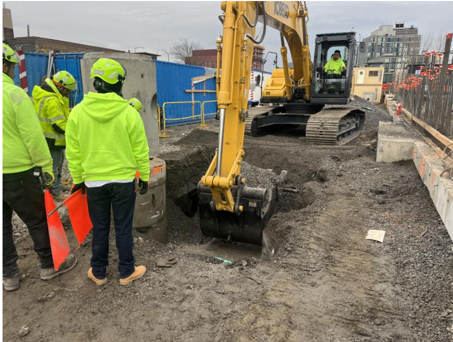
Photo 1: G&M excavating to install utilities in the northeastern part of Sackett Place within the SPW (facing south)
