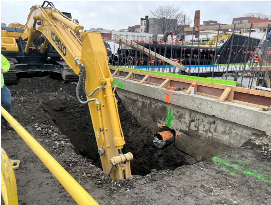
Photo 1: G&M excavating to install utilities in the southeastern part of Society Brooklyn within the SPW (facing south)
