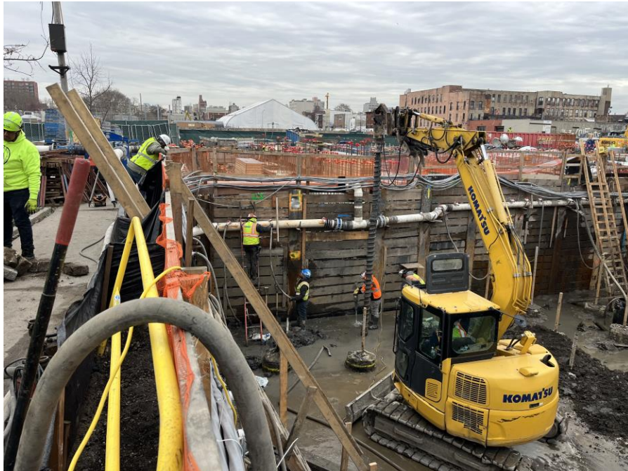
Photo 2: Kingdom installing dewatering wells for the dewatering system in the northern part of Society Brooklyn (facing east)
