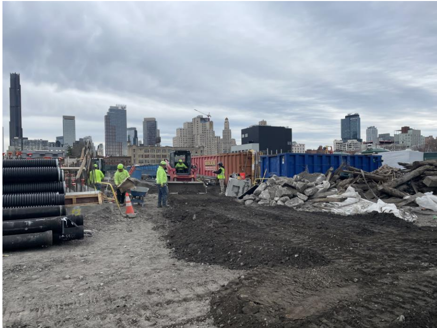
Photo 2: G&M backfilling around utilities in the southeastern part of Society Brooklyn (facing northeast)
