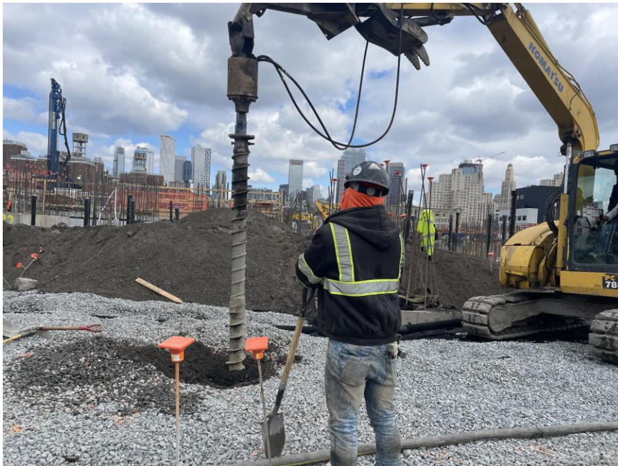
Photo 2: Kingdom installing post-treatment performance monitoring well in the central part of Sackett Place (facing northeast)
