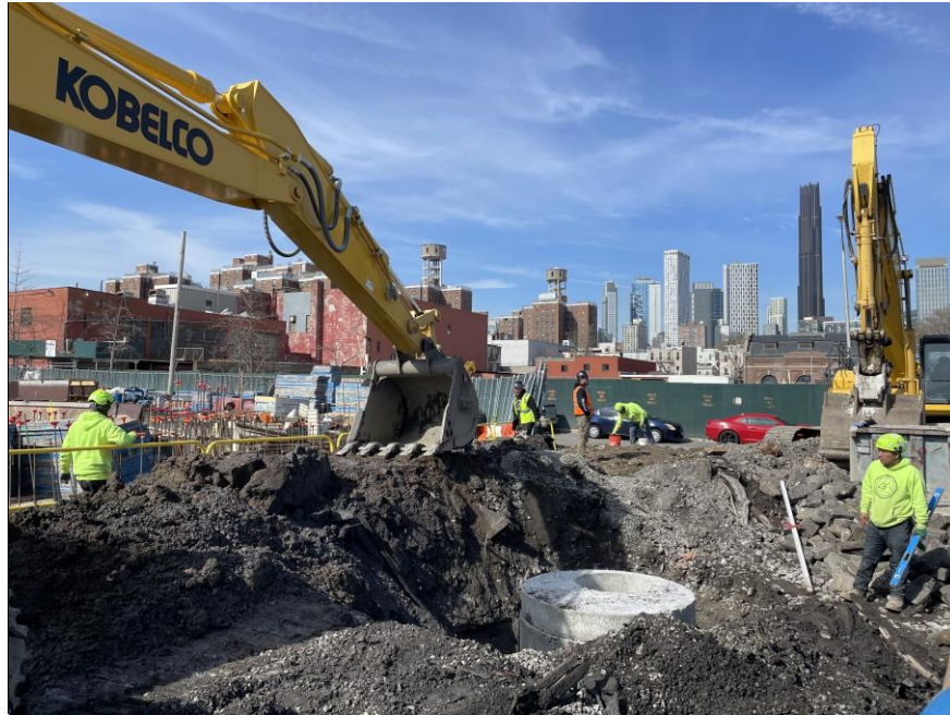
Photo 1: G&M excavating to install utilities in the eastern part of Society Brooklyn within the SPW (facing north)
