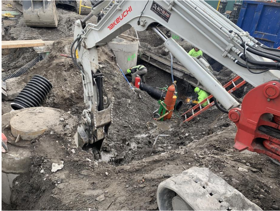
Photo 1: G&M excavating to install utilities in the southeastern part of Society Brooklyn within the SPW (facing east)
