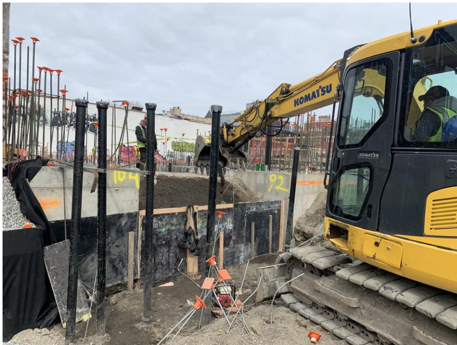
Photo 2: Kingdom backfilling around structural pile caps in the western part of Sackett Place (facing northwest)
