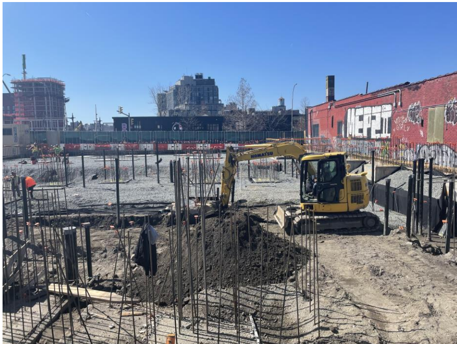
Photo 2: Kingdom backfilling around structural pile caps in the central part of Sackett Place (facing southwest)
