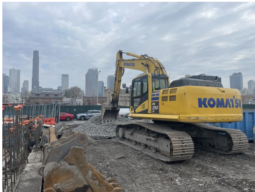
Photo 2: Kingdom placing 2.5-inch virgin quarry stone to repair the stabilized construction entrance in the northeastern part of Society Brooklyn (facing northeast)
