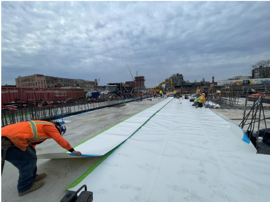
Photo 1: Kingdom installing a waterproofing/vapor barrier in the southeastern part of Society Brooklyn (facing south)
