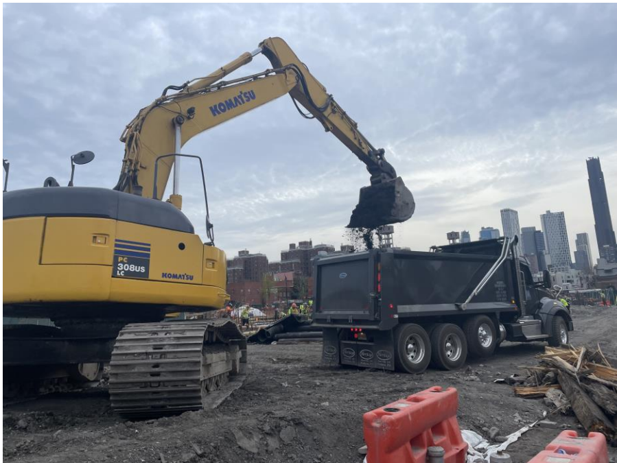
Photo 2: Kingdom exporting non-hazardous historic fill/soil in permitted tri-axle trucks in the northeastern part of Sackett Place (facing north)
