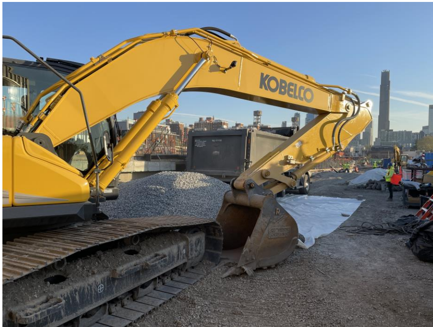
Photo 1: Kingdom importing ASTM #5 stone in the northeastern part of Sackett Place (facing northeast)
