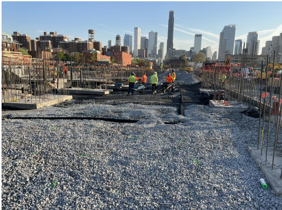
Photo 2: Kingdom installing SMD system components in the eastern part of Sackett Place (facing north)
